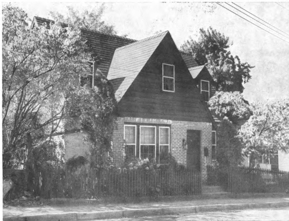
Fig 17. THE MANSE, HIGHLAND AVENUE MISSION
