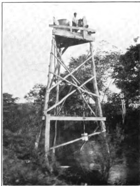
THE WATER SUPPLY
