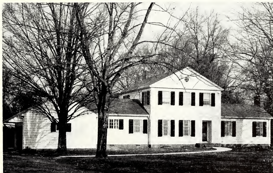
HAWFIELDS PRESBYTERIAN MANSE, COMPLETED OCTOBER, 1956
