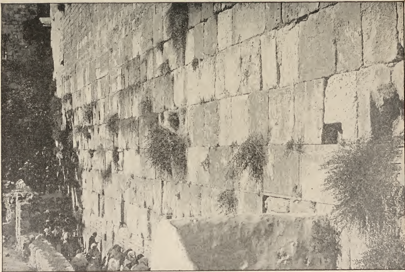
WAILING PLACE AND UPPER COURSES OF STONES IN WALL.
