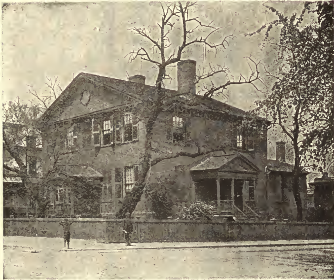
MARSHALL HOUSE, RICHMOND, VA.
