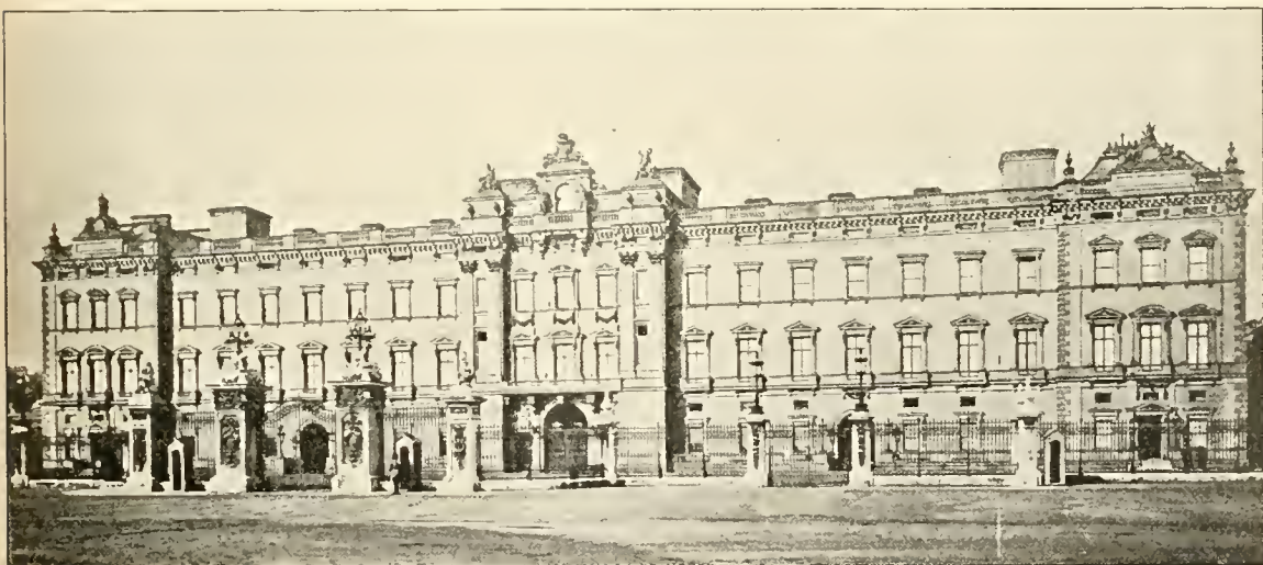
BUCKINGHAM PALACE, FRONT VIEW.
