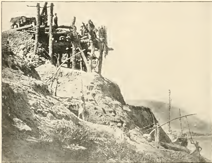
A SHADOF FOR RAISING WATER FROM THE NILE FOR IRRIGATION.
