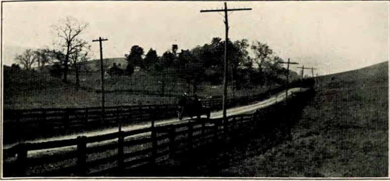
Photo by W. H. T. S. "FORT CHISWELL in the bluegrass uplands of the present county of Wythe."—P. 137. As the fort appears today.
