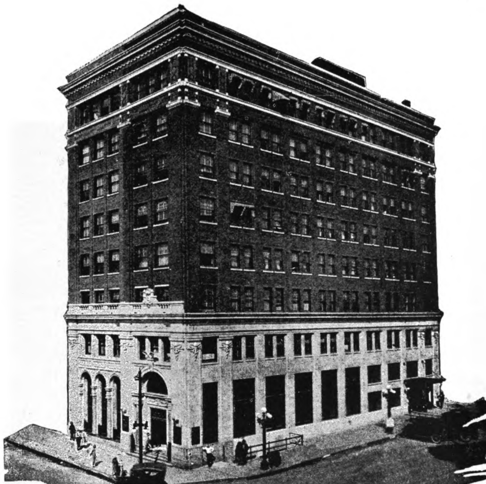
TEXARKANA NATIONAL BANK BUILDING, 1926-1927
