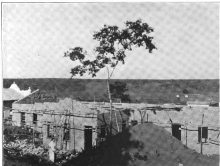
THE NEW HOSPITAL UNDER CONSTRUCTION AT PONTE NOVA The mound in the foreground is an ant hill (p. 300).
