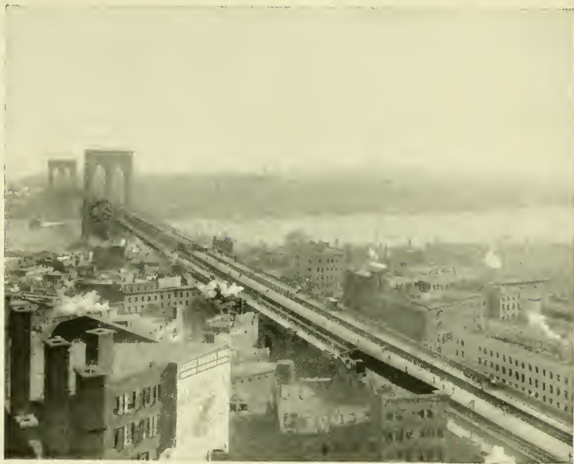
BROOKLYN BRIDGE FROM NEW YORK SIDE.
