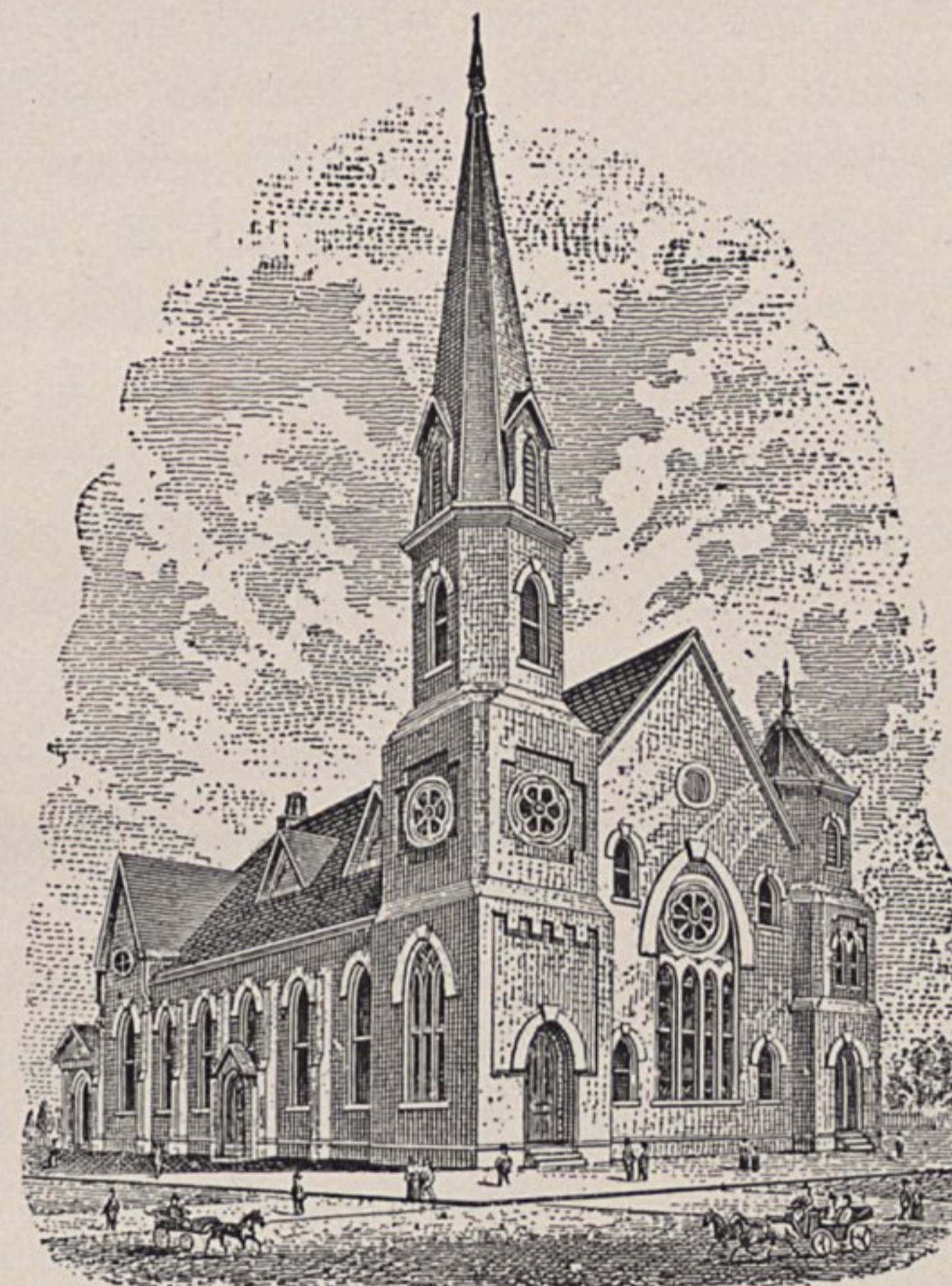
ST. ANDREWS CHURCH, PRESBYTERIAN. WILMINGTON, N. C.
