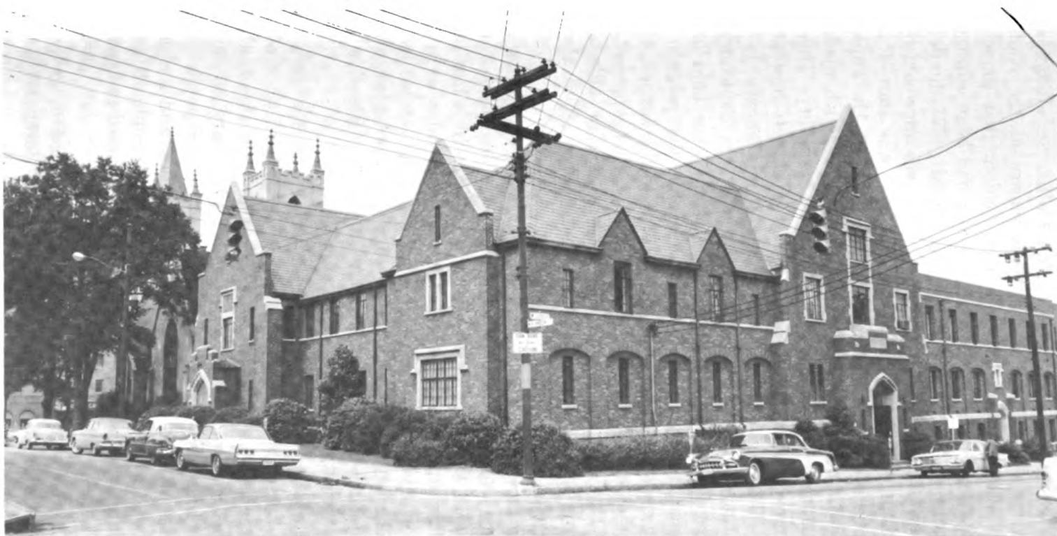
Sunday School from Coffee and Richardson Streets, showing the addition made in 1960.
