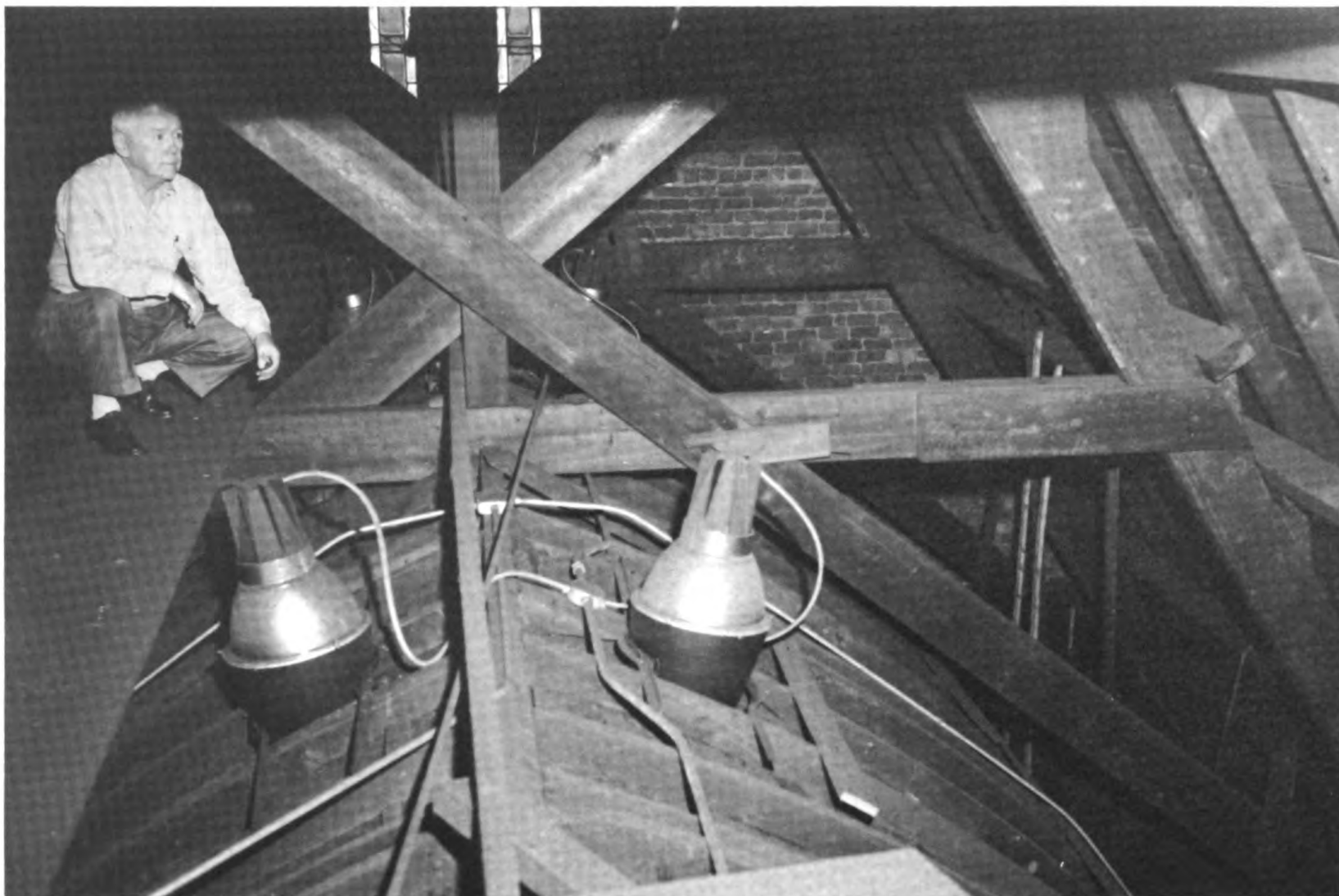
View of the roof and ceiling framing over the auditorium.
