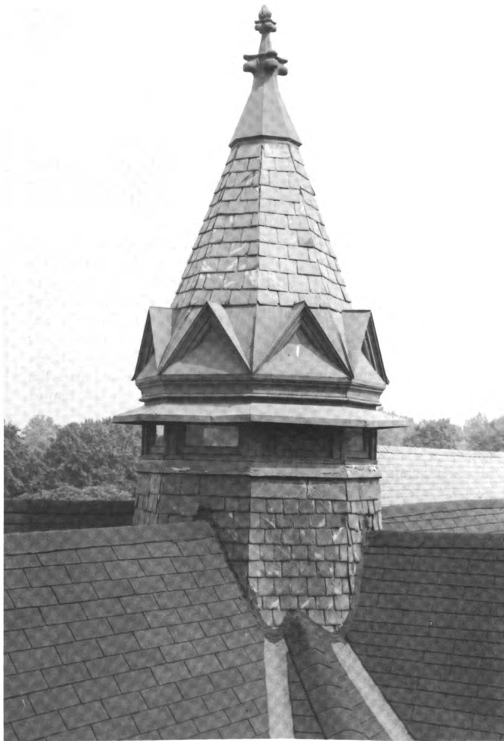
Tower for ventilation system, opening into the center of the auditorium. A panel with levers at the rear of the auditorium was connected by wires to the vents and could be opened or closed at will.
