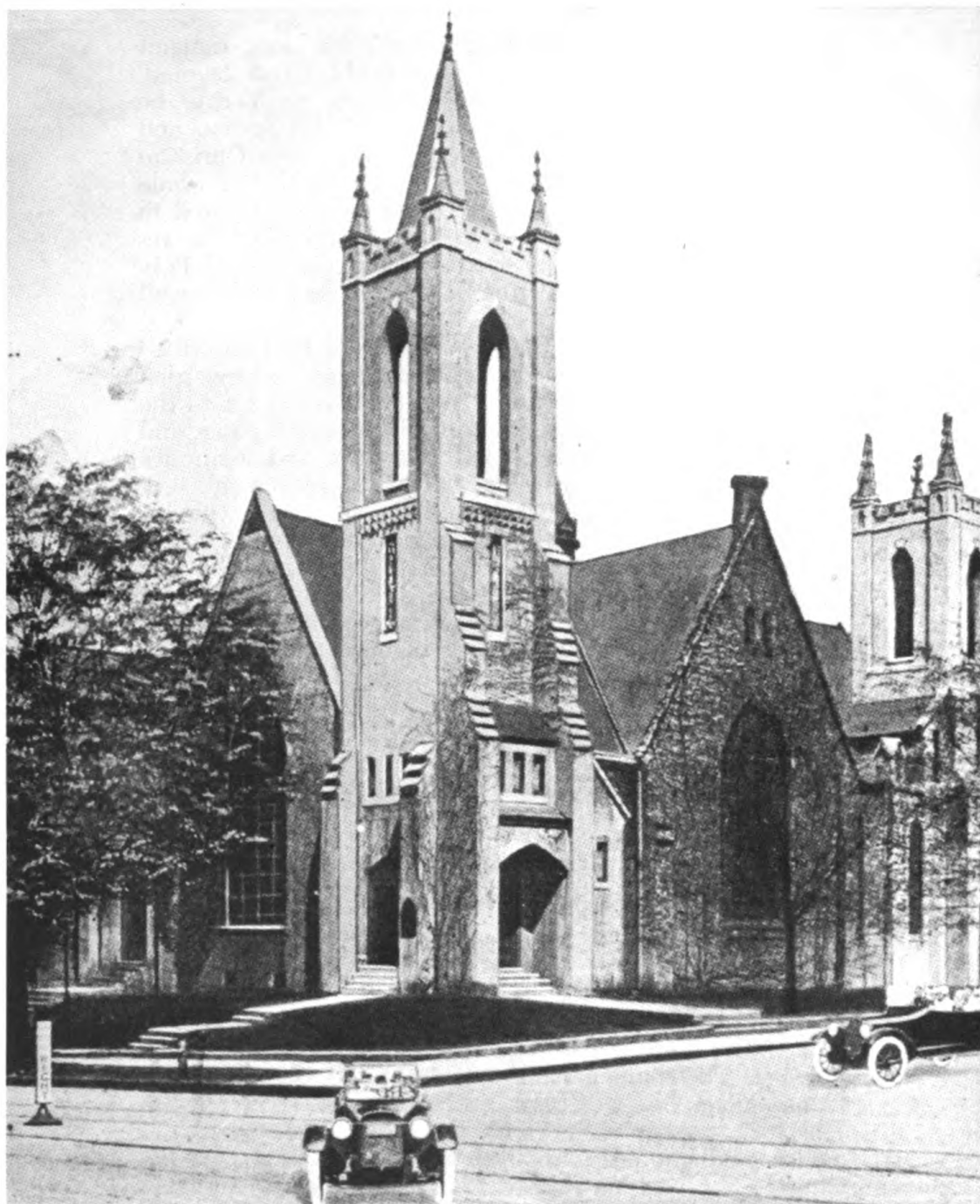
First Presbyterian Church from the corner of Washington and Richardson Streets, the first addition and the second tower added in 1912.
