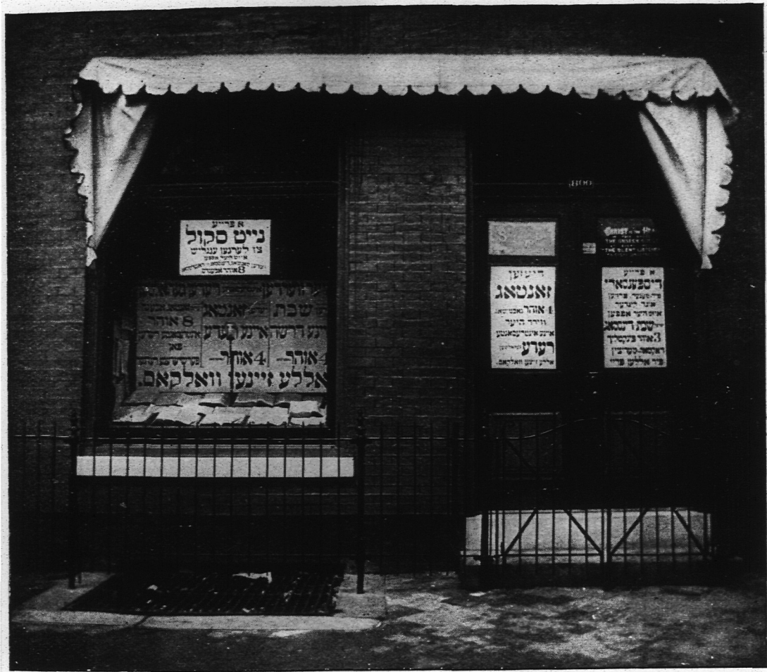
DOOR AND WINDOW IN THE MISSION BUILDING.
