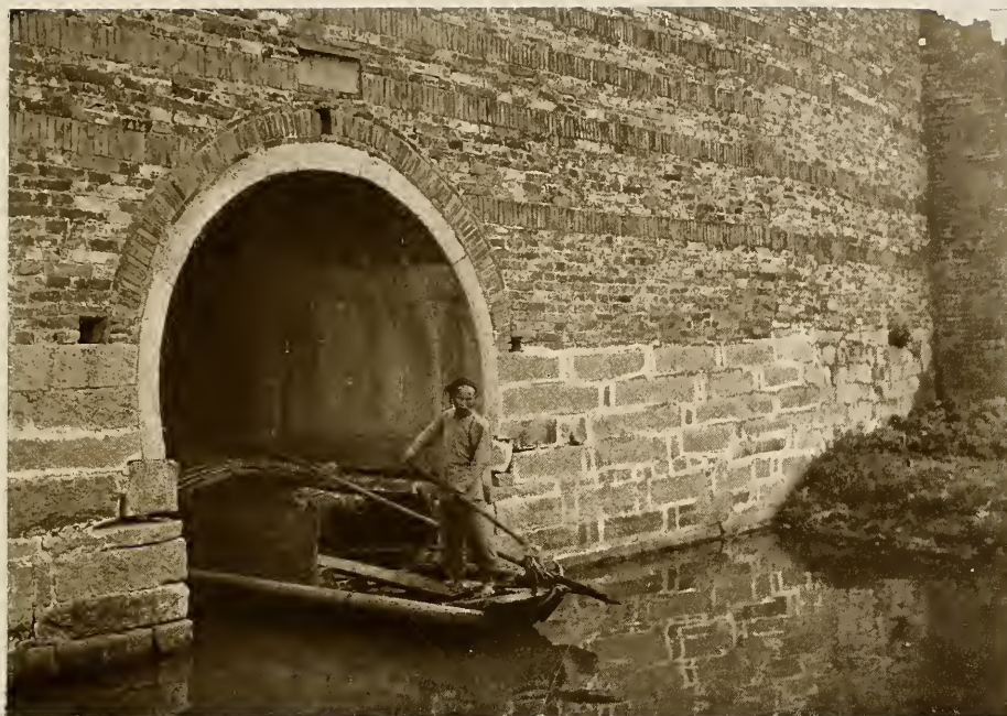
SUCHOW: ONE OF THE WATER GATES
