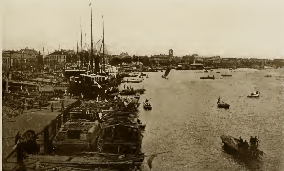
SHANGHAI: RIVER VIEW UP-STREAM
