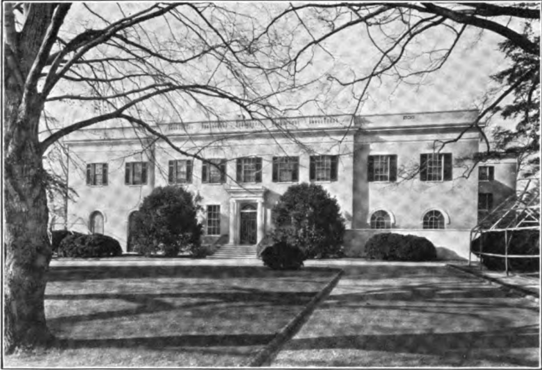
THE PRESENT "POINT BREEZE" The Manor House at "Bonaparte Park" (Photo by Mattie Edwards Hewitt, N. Y.)
