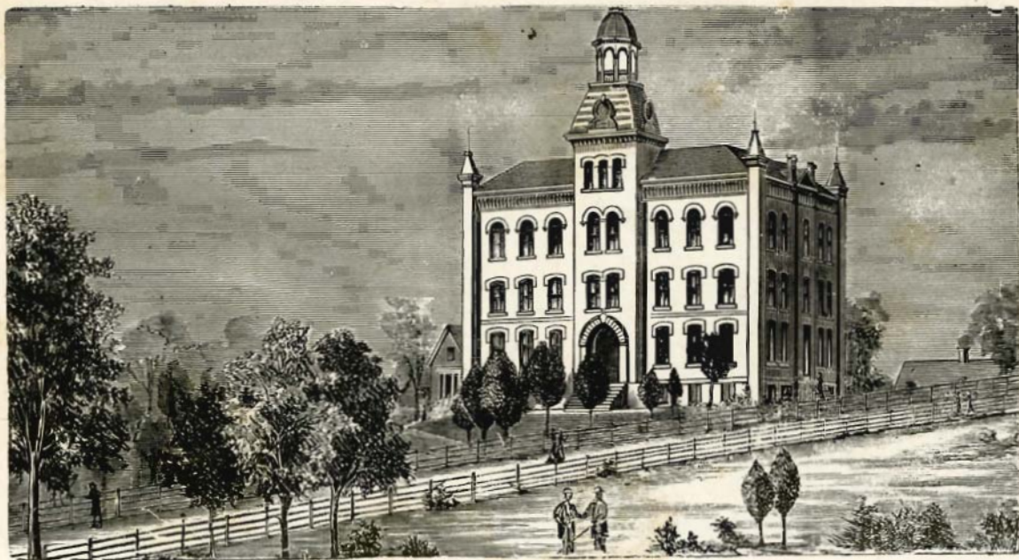
FIRST COLLEGE BUILDING, DEDICATED IN 1876. BURNED IN 1894.
