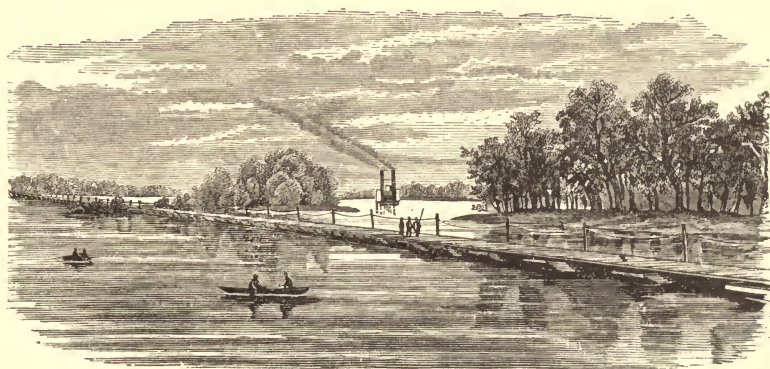
PONTOON BRIDGE AT PADUCAH.
