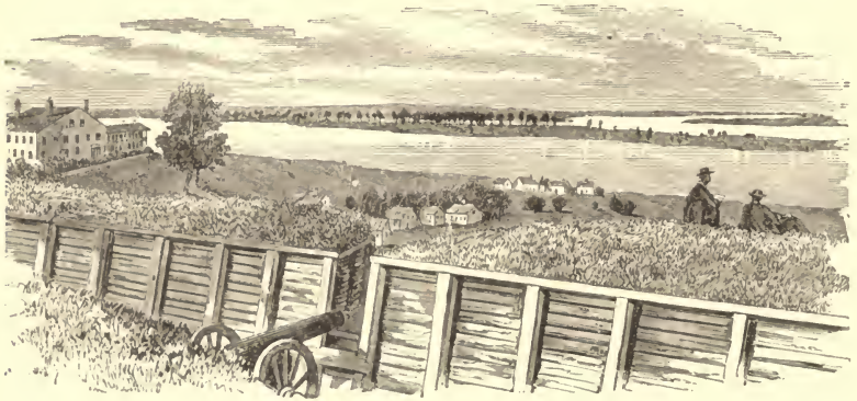
VIEW SHOWING THE SITE OF THE CANAL.
