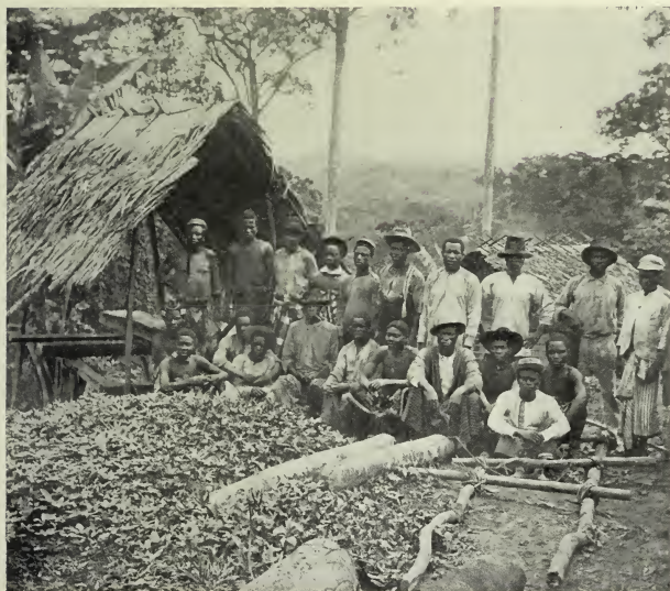
PIT-SAW AT EFULEN AND WORKMEN FROM SEVERAL TRIBES.
