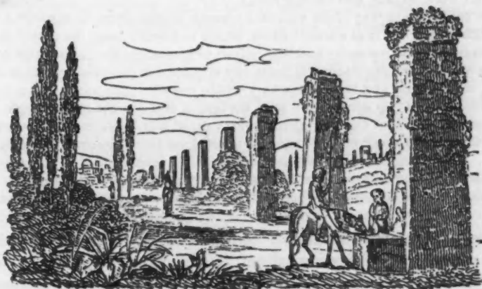
Sooteray, or substitute for Aqueduct.
