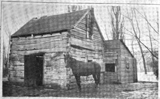
JOHN FRASER'S LOG HOUSE 1868
