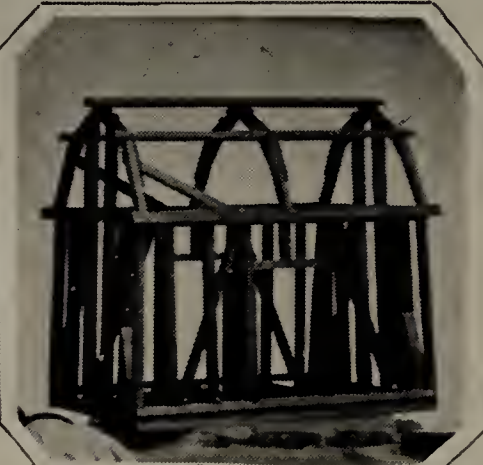
ROOF TRUSS OF JACOB H. F.
