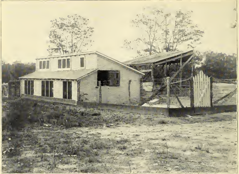
THE HEN HOUSE; OPEN FRONT, SEMI-MONITOR ROOF
