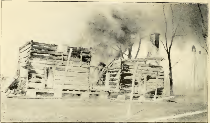
THE FLAMES CONSUMING THE OLD FARM HOUSE, LOOKING NORTHEAST.
