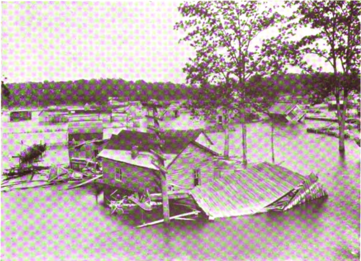
"THE HOUSES SLIPPED INTO THE STREAM"
