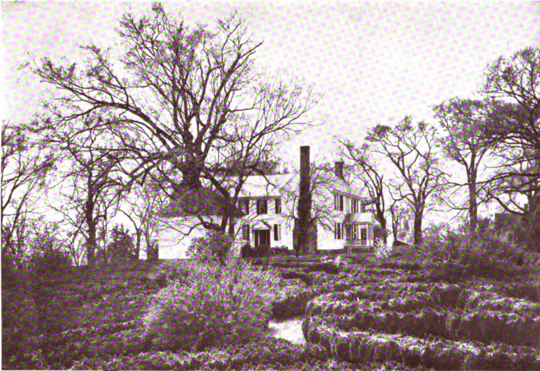
TUCKAHOE, ACROSS THE JAMES RIVER FROM WARWICK, VIRGINIA
