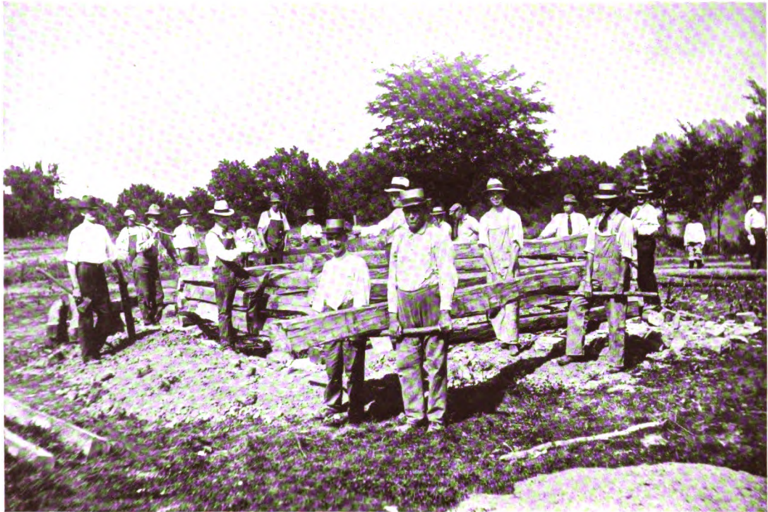
REBUILDING ONE OF THE OLD LOG CABINS, NEW SALEM, ILLINOIS
