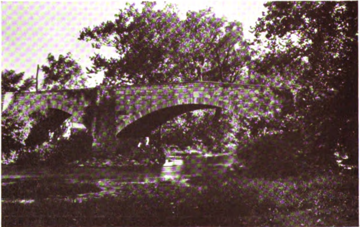
"ONE OF THOSE SOLID HIGHWAY BRIDGES"
