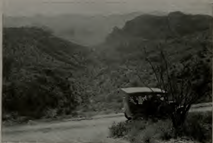
ROOSEVELT ROAD, ARIZONA
