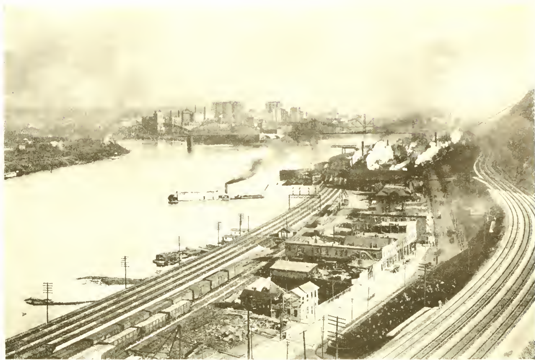
OHIO, ALLEGHENY AND MONONGAHELA RIVERS, PITTSBURGH, FROM SOUTH SIDE Photo by John C. Bragden
