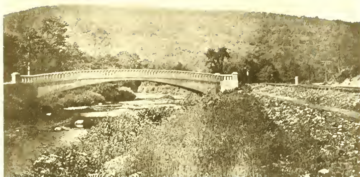
HIGHWAY BRIDGE ACROSS ELK CREEK, NEAR RIDGWAY Photo by State Highway Department
