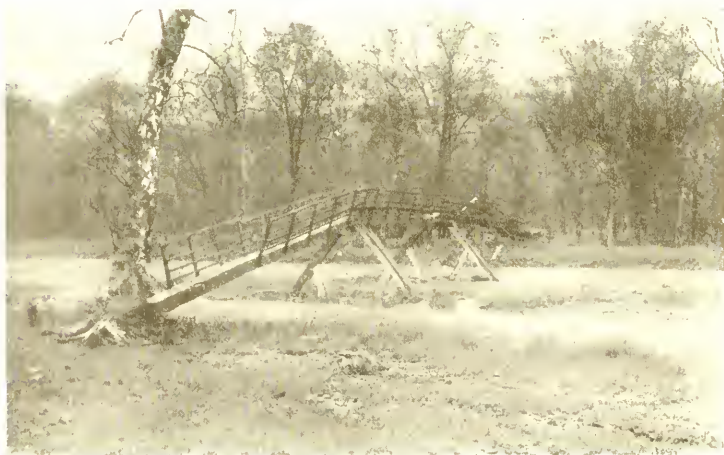
WEBSTER MILLS BRIDGE, FULTON COUNTY Photo by State Highway Department
