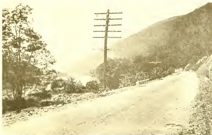
ALONG THE JUNIATA Photo by State Highway Department
