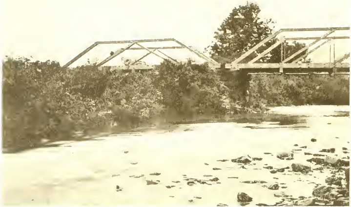
LITTLE BROKENSTRAW CREEK, WARREN COUNTY Photo by State Highway Department
