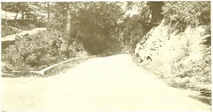
PENETRATION ROAD IN MERCER COUNTY Photo by State Highway Department
