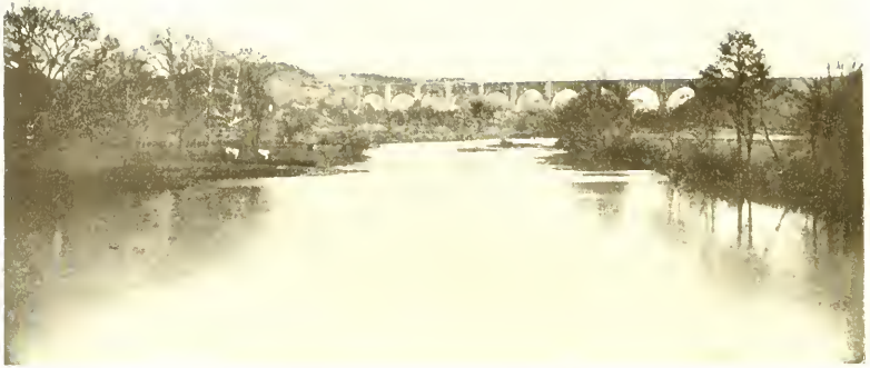
NICHOLSON VIADUCT, WYOMING COUNTY Photo by State Highway Department
