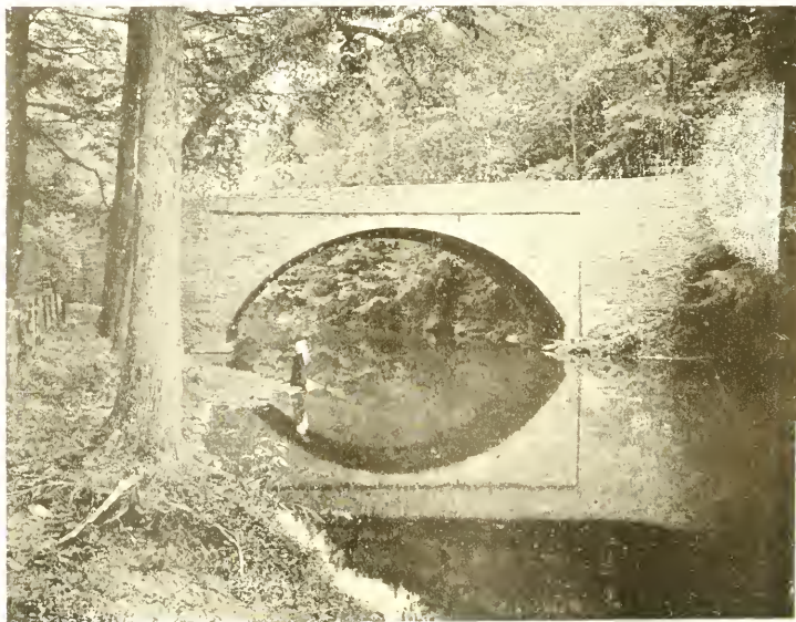
VALLEY GREEN BRIDGE, WISSAHICKON DRIVE Photo by J. Horace McFarland Company
