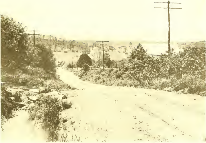
IN VENANGO COUNTY Photo by State Highway Department
