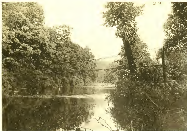
SUSPENSION BRIDGE ON FOUR MILE RUN NEAR LIGONIER Photo by W. T. Brown
