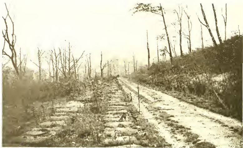
STONE SLEEPERS, FOURTEEN MILE LEVEL, OLD PORTAGE RAILROAD, LOOKING TOWARD MINERAL POINT
