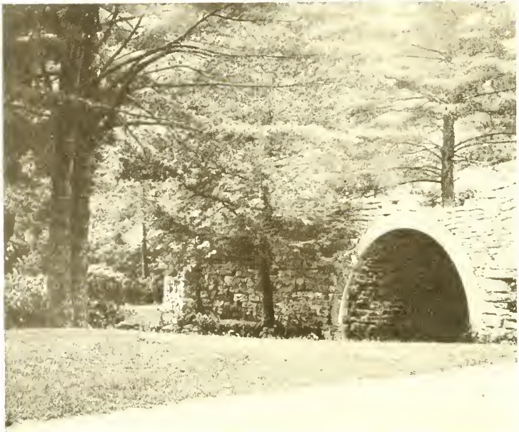
OLD VIADUCT ACROSS TOMS CREEK ON TAPEWORM RAILROAD Photo by State Department of Forestry
