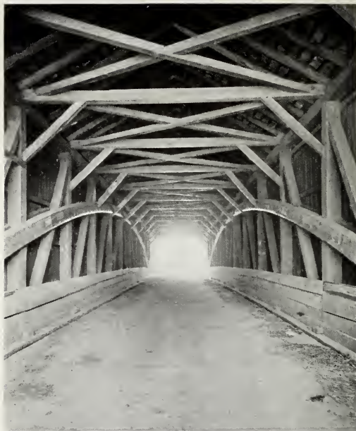
INTERIOR OF A COVERED TURNPIKE BRIDGE
