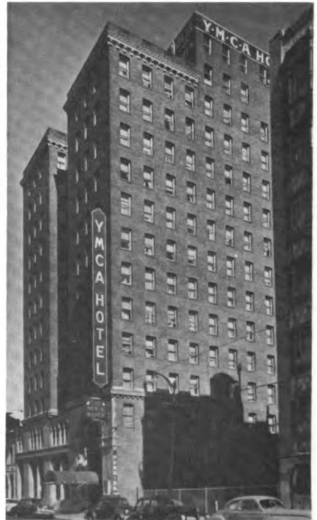
THE Y.M.C.A. HOTEL AT 351 TURK STREET Charles P. Taft, son of President Taft, sealed its cornerstone on Jan. 17, 1929, twenty years after the Y.M.C.A. building at 220 Golden Gate Avenue had been dedicated by his father.
