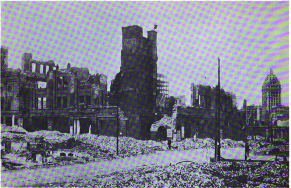
RUINS OF THE MASON-ELLIS BUILDING Destroyed by the 1906 San Francisco earthquake only three years after its dedication by President Theodore Roosevelt in 1903.
