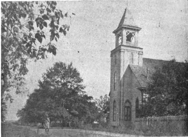
PRESBYTERIAN CHURCH, CAMDEN, ALABAMA, About 1894
