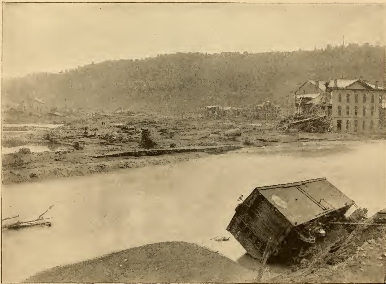
TRACK OF THE FLOOD.
