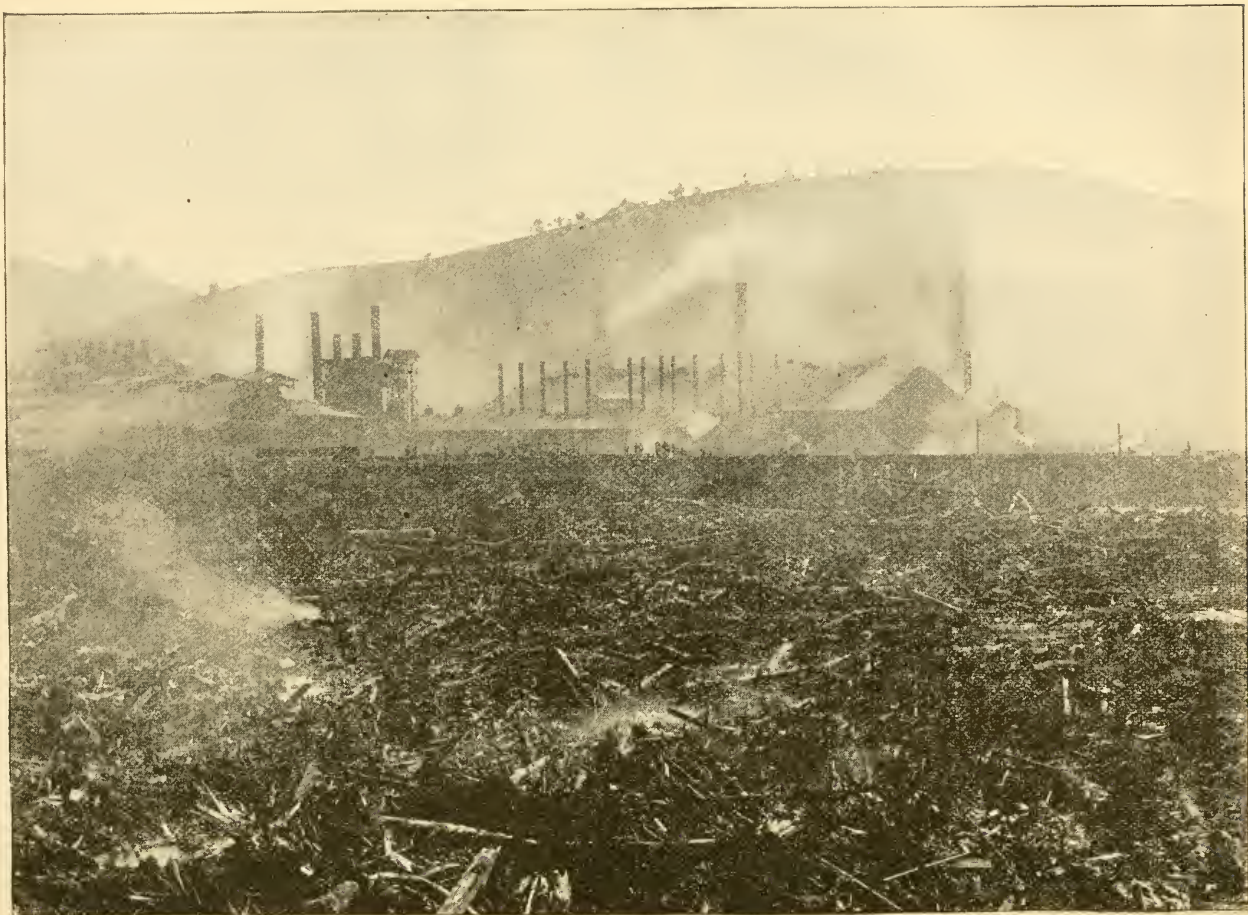
DEBRIS ABOVE THE BRIDGE; CAMBRIA LOWER WORKS IN THE DISTANCE.
