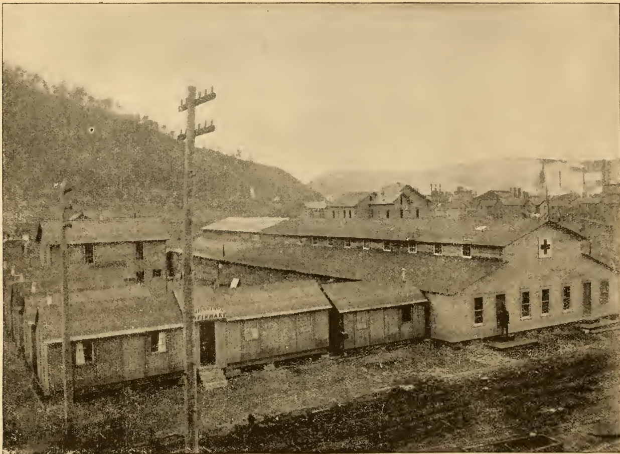
RED CROSS BUILDINGS ON SITE OF JUDGE POTTS'S FORMER RESIDENCE.
