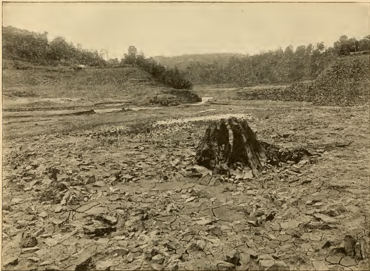
VIEW OF THE BROKEN DAM, LOOKING FROM THE LAKE BASIN.
